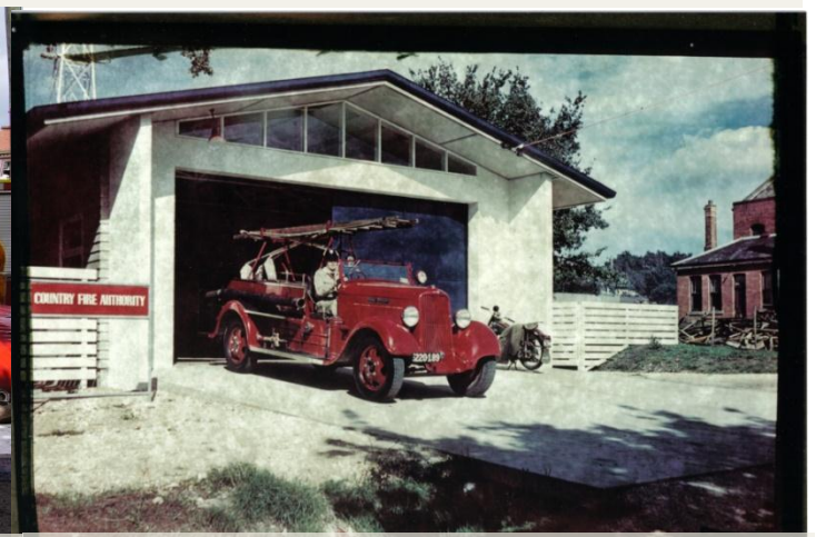
New Fire Station circa 1955 – Note the rubble from the original fire station demolition in the background.
