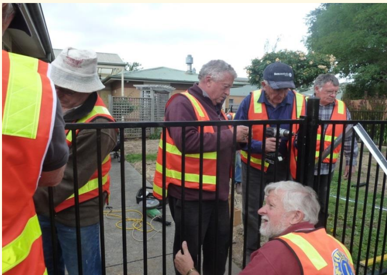
Lions at work fitting one of the security gates
