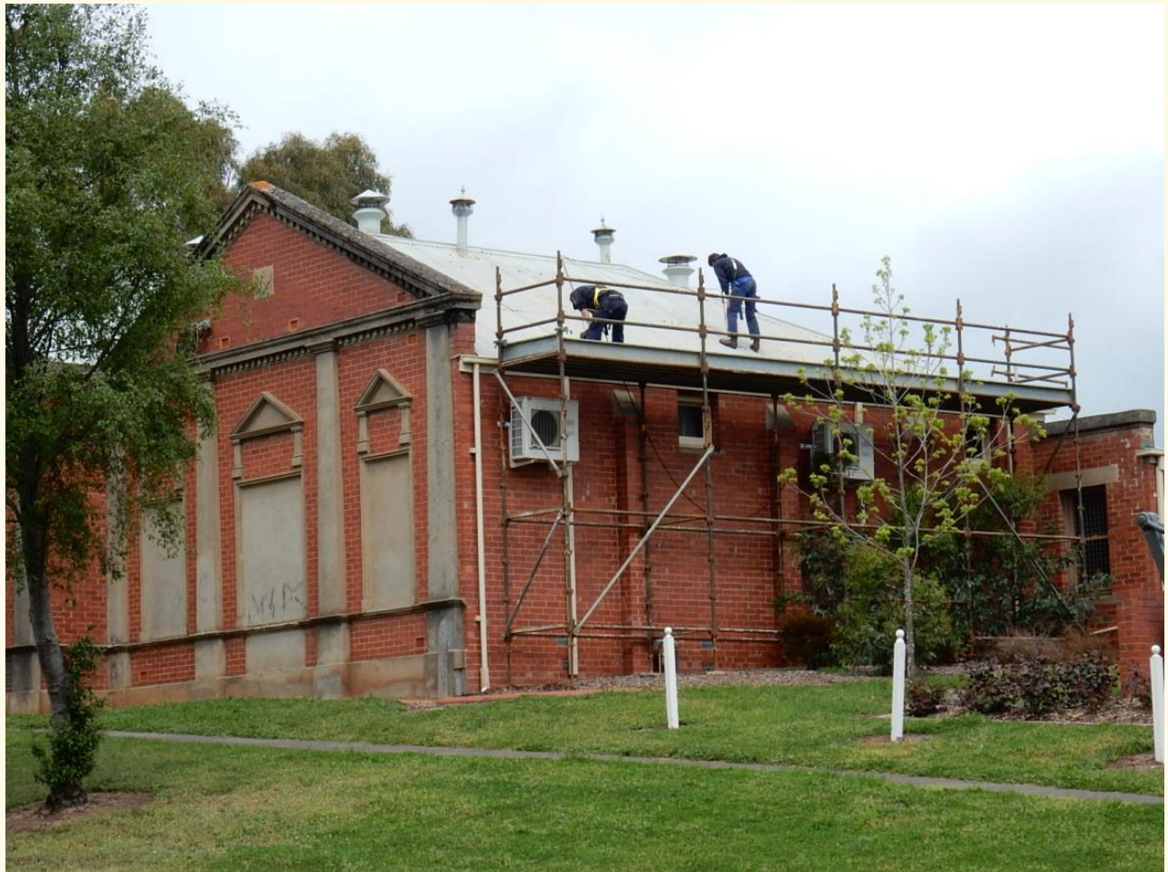
Photo: Roof repairers working of the Masonic Centre roof.
