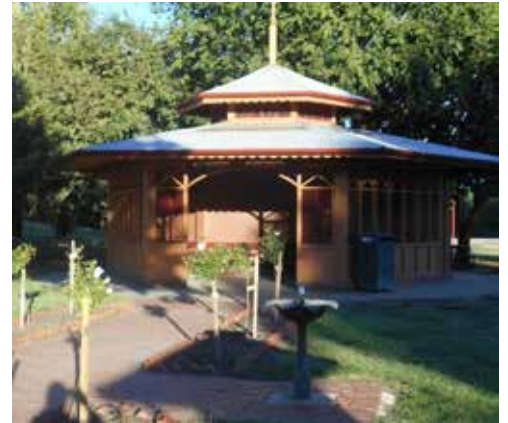
Rotunda to be converted and retained
