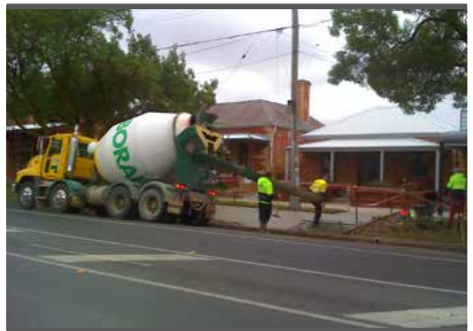
The concrete truck arrives three days later on 10 April
