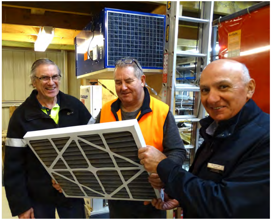
Checking dust on a filter taken from one of the units shown at the rear of the group are (L to R) Chris Kruger, Mens' Shed President Graham Perkins, and Ian Corcoran.
